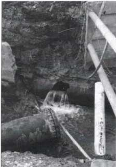
Existing 42-inch main (on top)
